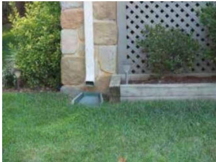
Simple Rooftop Disconnection – (Photo: Center for Watershed Protection)
